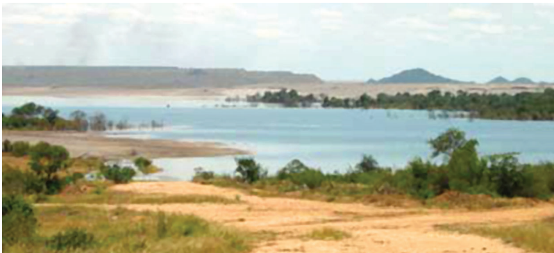
The Foskor tailings dam
