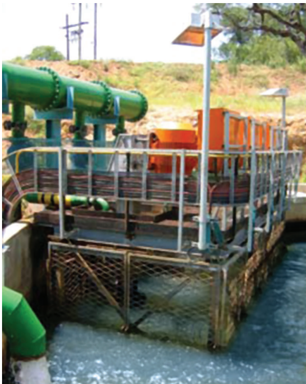
Three Warman 100RV vertical spindle pumps pumping in parallel to the Van Ryssen dam
