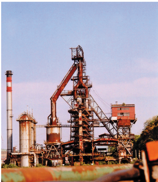
A blast furnace and surroundings. The blast furnace is inside the central girderwork.
