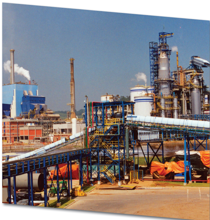
A chemical plant
